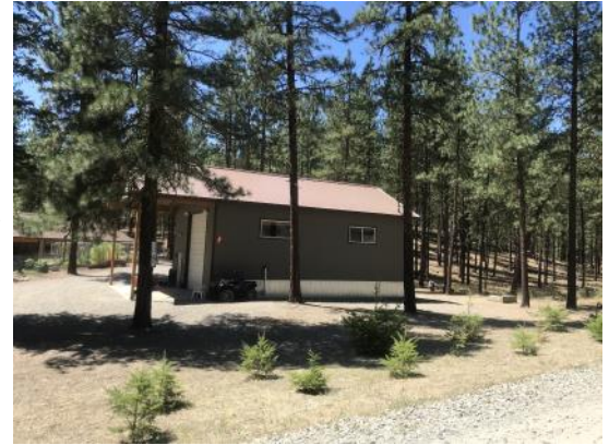
Home with defensible space and fire resistant roof and siding.
